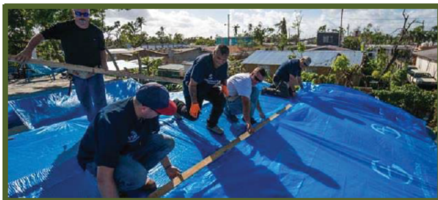
Figure 3: Relief Workers Installing Tarp on Damaged Home, December 2017
